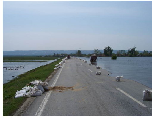
Figure 5. Dyke cracking prevention with used belt conveyors to realize the swirl water dispersion.
