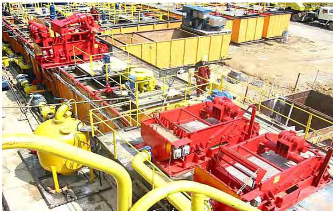
Figure 2. Produced water storage tanks [5].
