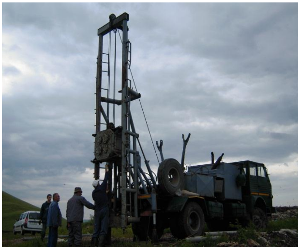
c. Start drilling
