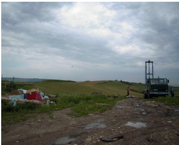
a. Placing the drill plant
